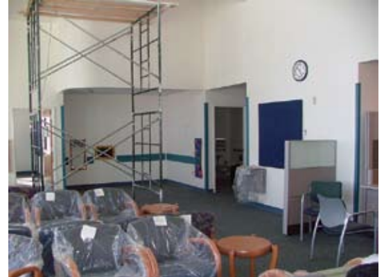
Hooper Bay SRC nears completion.
