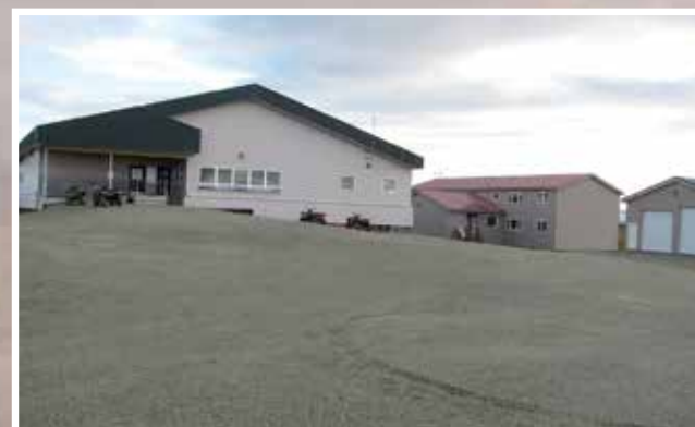
Thanks to Nunakauyak Traditional Council, the Toksook Bay Subregional Clinic got a load of gravel in their front lot. This will improve air quality in the community by controlling dust.
